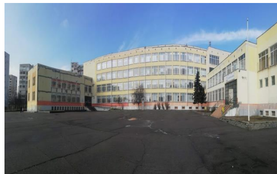
Source: NTEF archives, Project name: "Improving the energy efficiency of 79 Indira Gandhi High School, Lyulin district"
