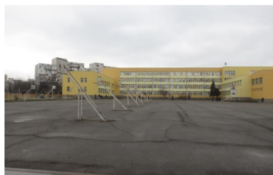
Source: NTEF archives, Project name: "Improving the energy efficiency of 79 Indira Gandhi High School, Lyulin district"
